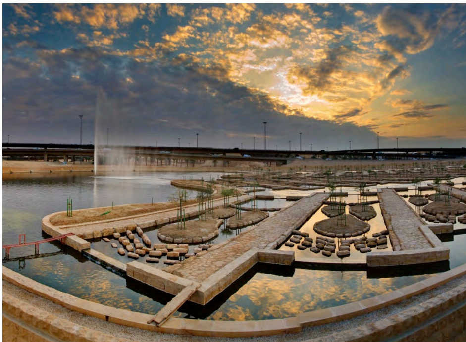
Figure 14. The Wadi Hanifa project successful in providing water treatment while creating a one-of-a-kind natural facility and open-space public attraction (Source: Aga Khan Award for Architecture)
