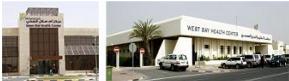
Figure 33: On the left New VS. Old Primary Healthcare Center Design to the Right (Source: Primary Health Care Corporation, 2017)
