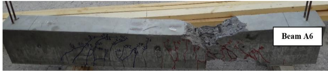
Figure 41. Beam A6 (Compression shear failure)
