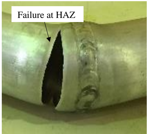
(c): V-welded pipe fracture in lower side
