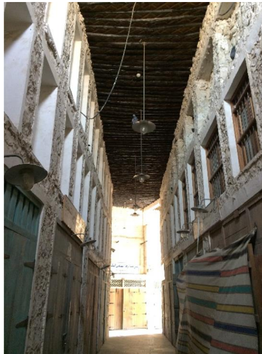
Figure 2 Wooden Roof (source: Author)
