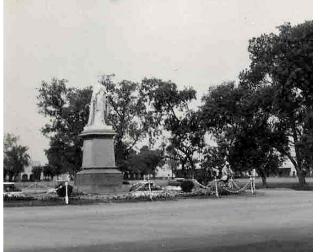
Figure 18 Queen Victoria's Statue, Rawalpindi, 1939(Source: https://Defence.Pk )
