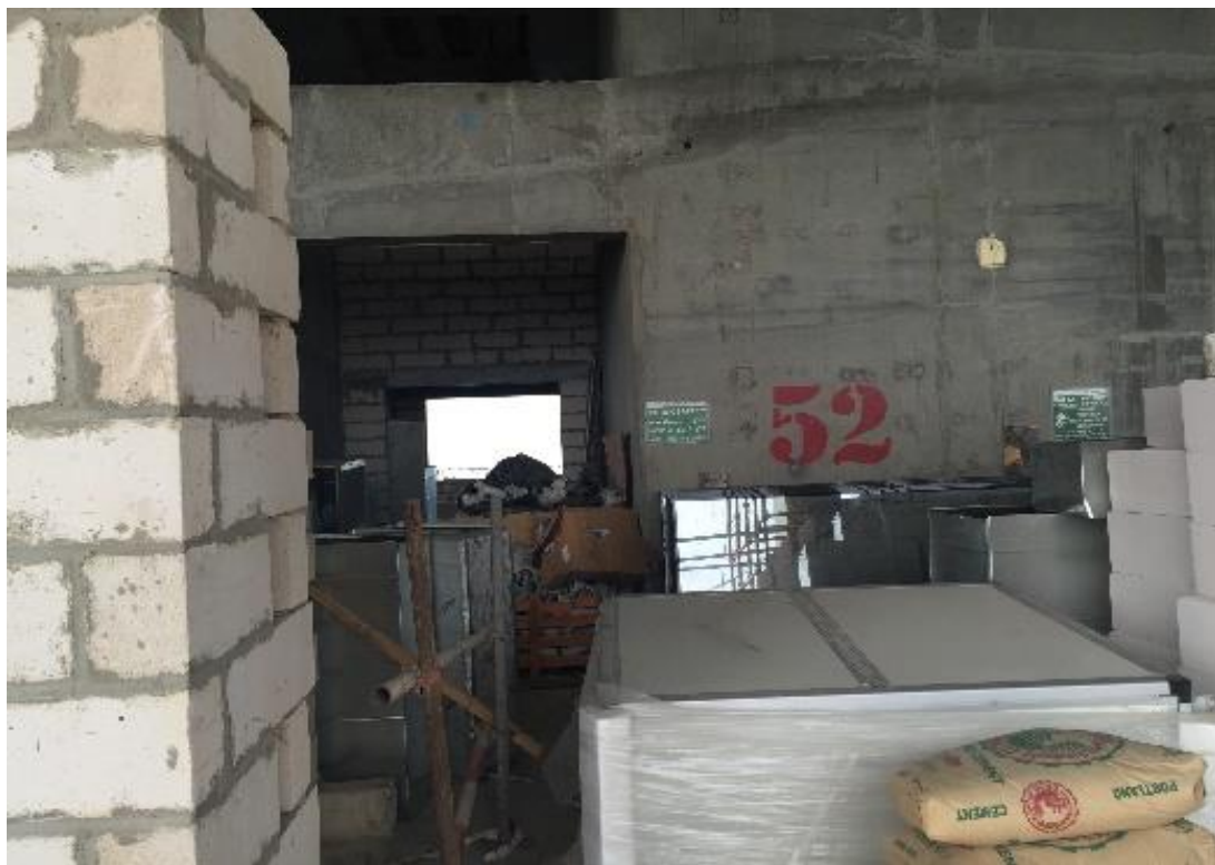
Figure 22. Floor 52 during Construction stage
