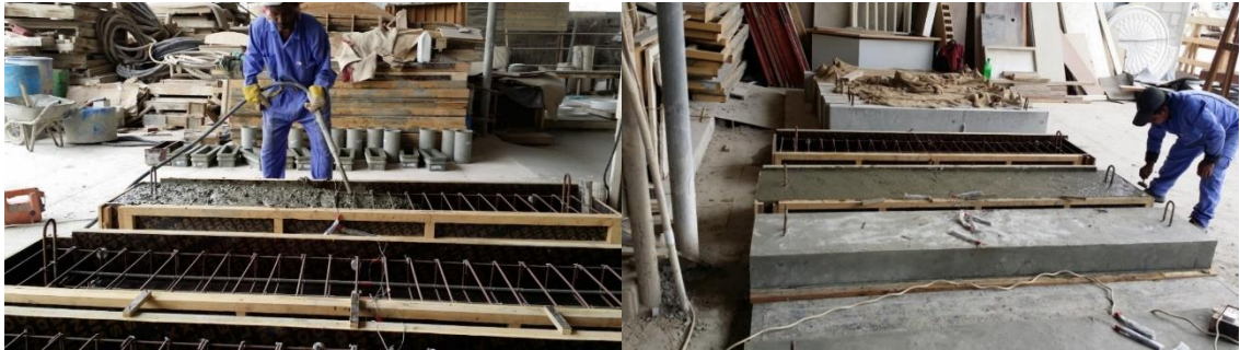
c) Using Vibrator Machine
