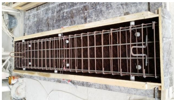
c) Cage inside the Mold
