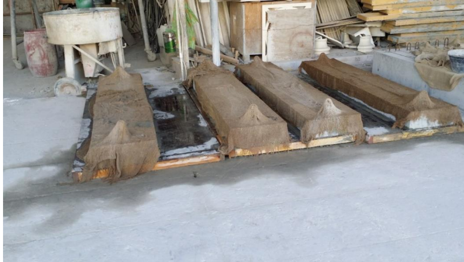
Figure 16. Curing of One-Way Concrete Slabs
