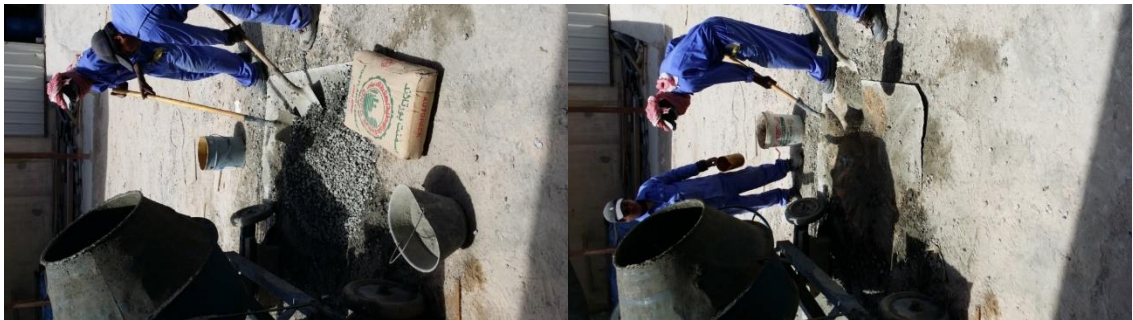
c) Putting Coarse Aggregate
