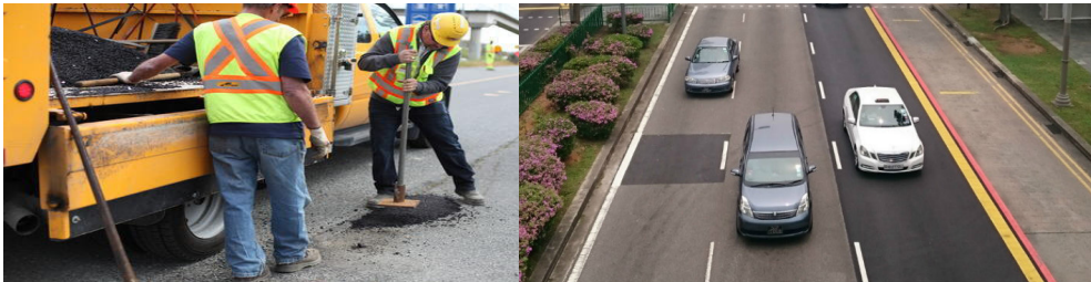
Figure 6: Prompt road maintenance on site
