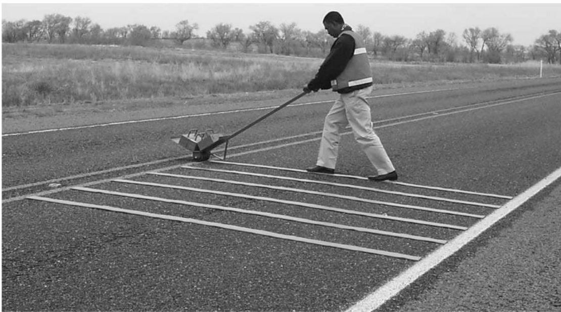
Figure 9. The installation of the rumble strips (Fontaine & Carlson, 2001).
