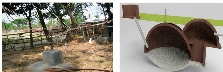
Figure 2. A Domestic Fixed Dome Biogas Plant Constructed from Brick, Sand and Cement (Left) and a Simulated Side View of an AD Plant (Right) [24].
