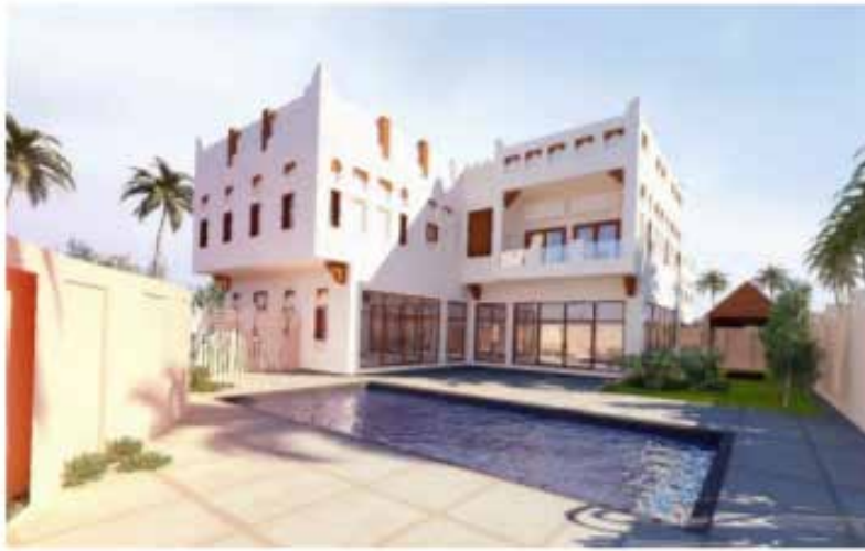
Figure 02: Typical Khaleeji home, located in Doha, Qatar is used for experimental study. Image courtesy of MZ & Partners (2017).
