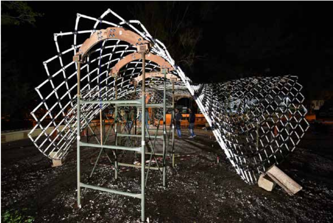
Figure 07: Assembly process, Scaffolding and digitally fabricated formwork.
