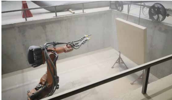
Figure 14: Robotic industrial arm sand blasting shell cassettes for correct finish texture.
