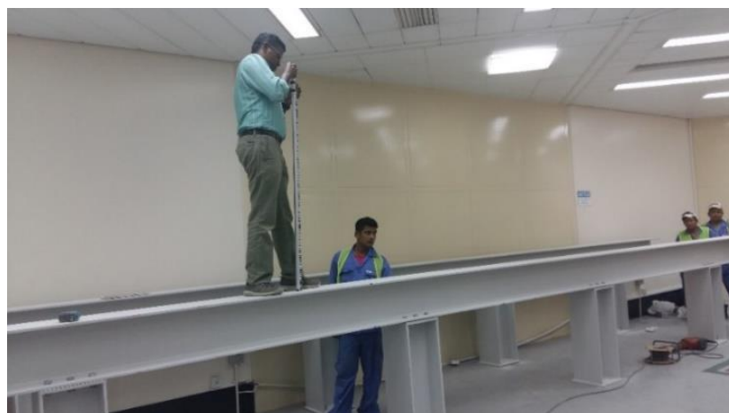
Figure 102. Leveling of the Steel I-beam
