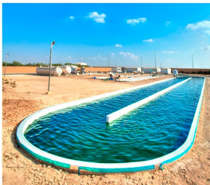
Figure 3. The semi-buried raceway used for microalgae culture in Qatar [84].
