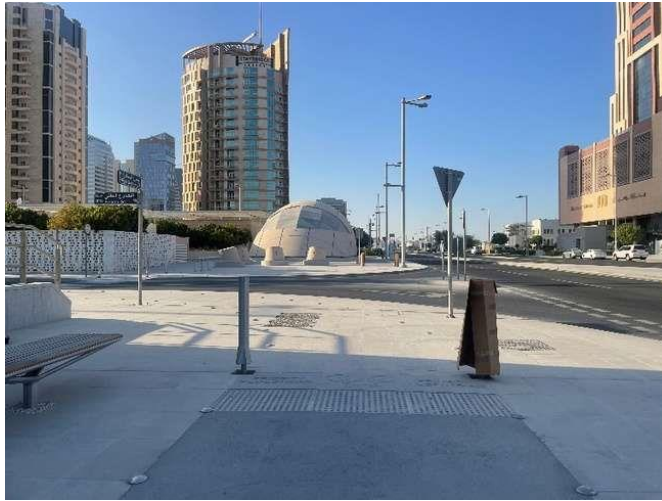
Figure 79. Unclear pathways on primary road (Source: Author)
