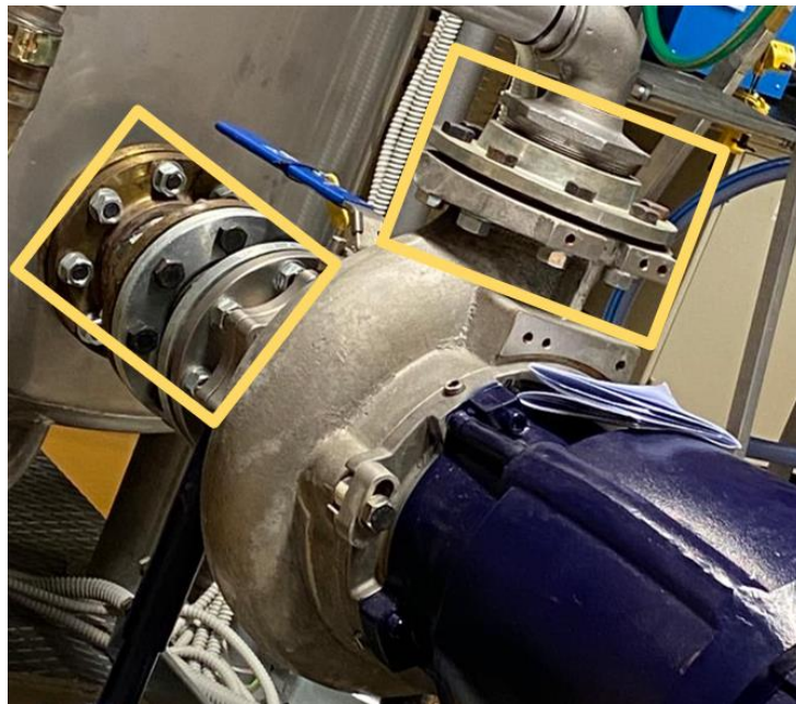
Figure 9: Flanges attached to the tank
