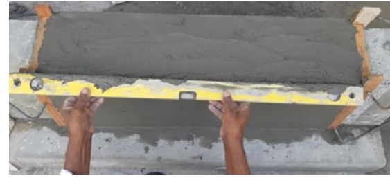
(b) Application of final mortar layer and surface finishing
