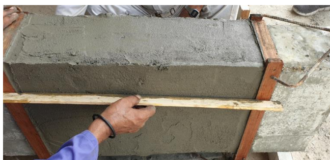
(a) Application of first mortar layer
