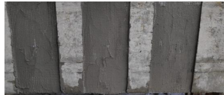
(b) Steel fabrics being installed and impregnated with the matrix
