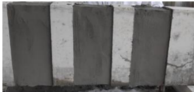
(a) Application of geo-mortar in the prepared groove
