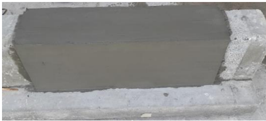
(c) Final finished surface
