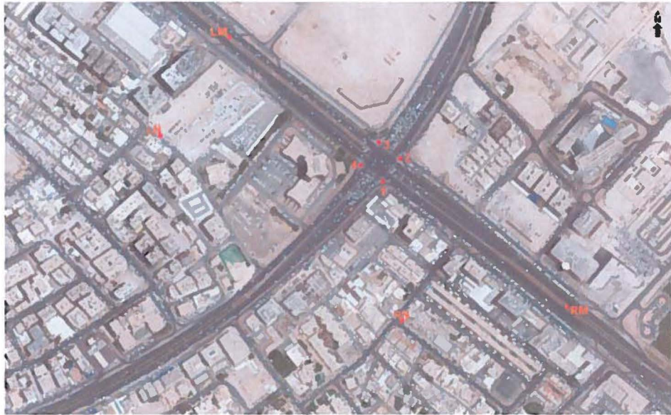
Figure 16. Intersection nearby Toyota Tower (E) with 2 – 250m proximity points (RM and LM) and neighboring points away from the main road (RN and LM). Google Earth, 2012
