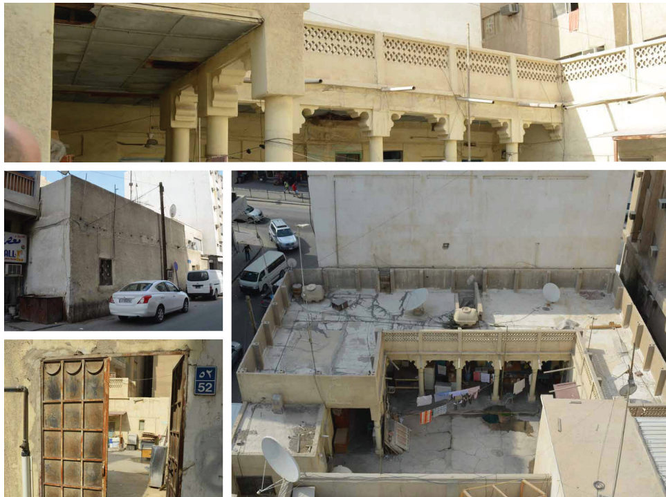
Figure 8. Recent situation of an old courtyard house in Doha. Source (PEO 2015).
