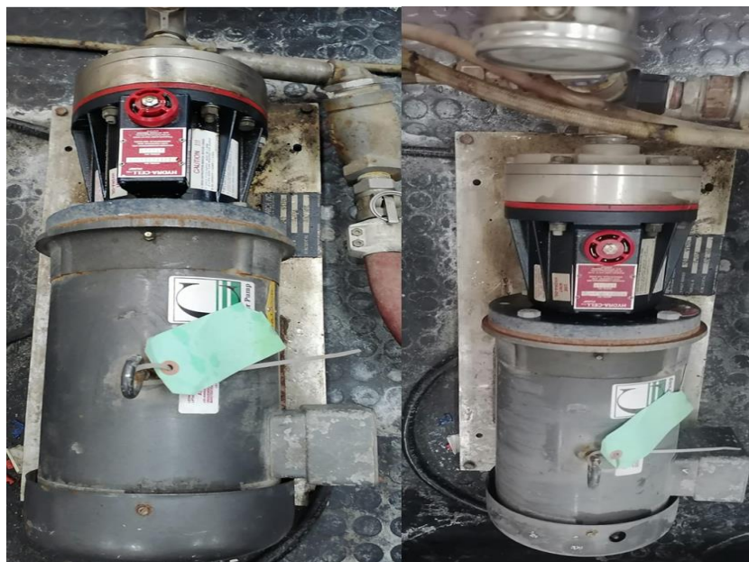
Figure 11: The feed pump in VSEP.
