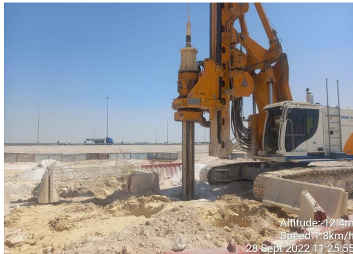
Fig. 2a: Photograph of BAUER BG-11 Piling Rig in Action
