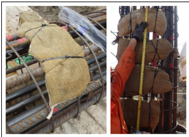
Figure 17. Site photos of sandbags.
