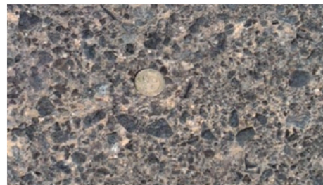
d) Salwa road (8 years with NMAS of 19 mm with MTD of 2.92)
