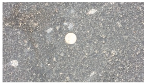
b) Rawdat Al Rashed road (1 year with NMAS of 19 mm with MTD of 0.95)
