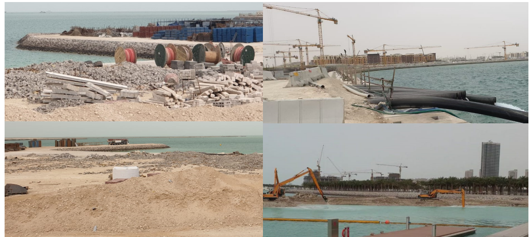
Figure 10. Ongoing coastal construction in Lusail City.
