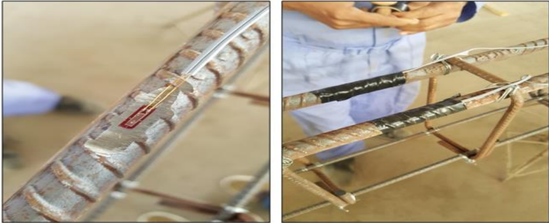
Figure 3.9 Fixing of Steel Strain Gauges
