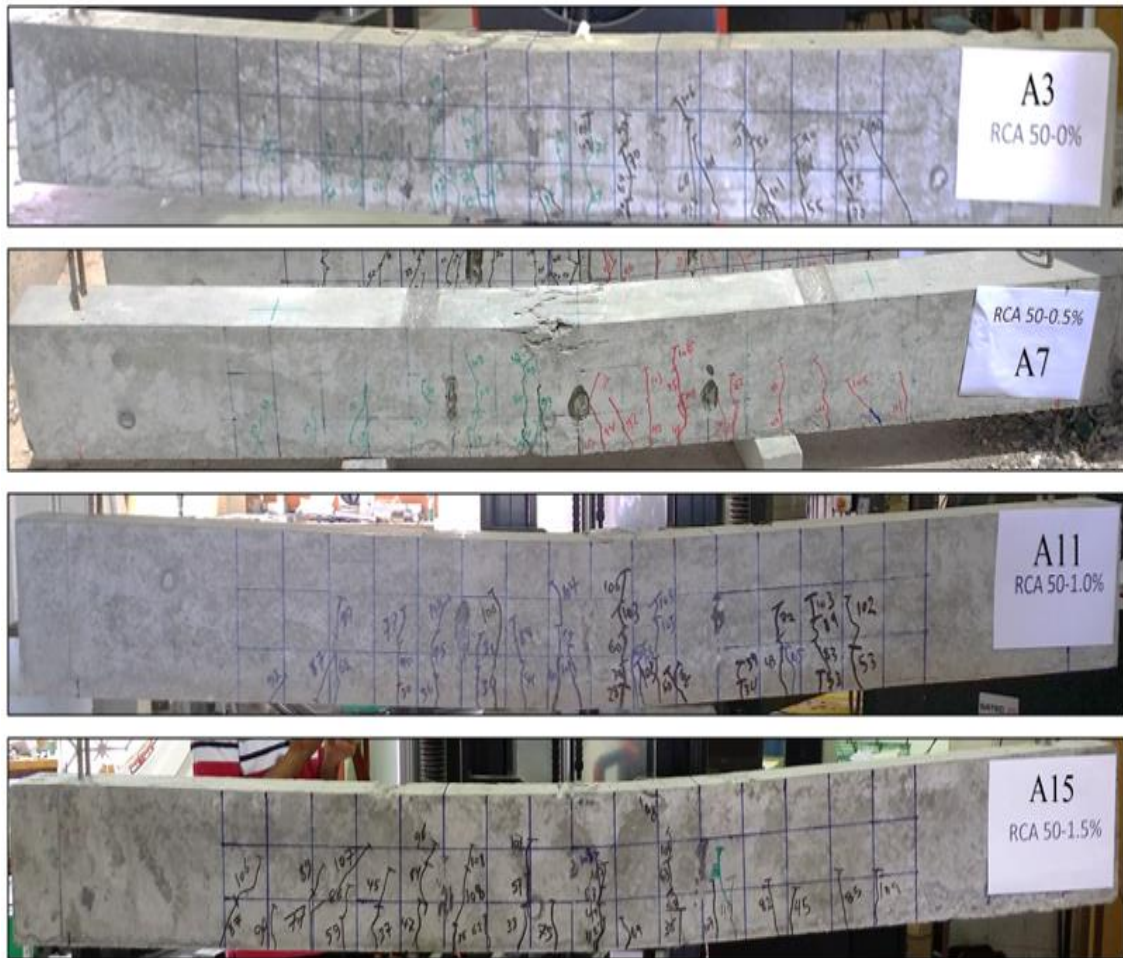
Figure 4.62 Crack Pattern in Test Beams A3, A7, A11 and A15
