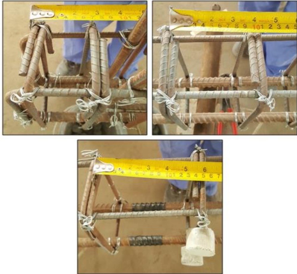
Figure 3.7 Stirrups Distribution
