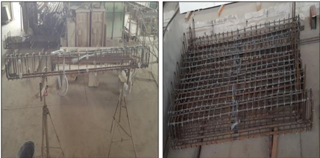
Figure 3.6 Steel Cages
