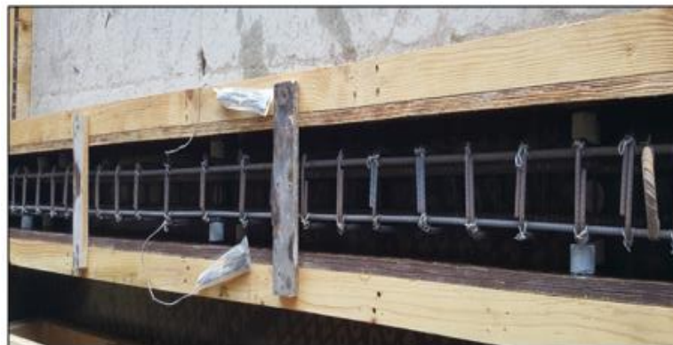
Figure 3.8 Framework and Steel Cage with Cover Spacer
