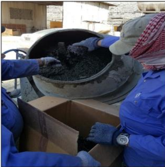
Figure 3.13 Adding BMF Inside the Concrete Mechanical Mixer
