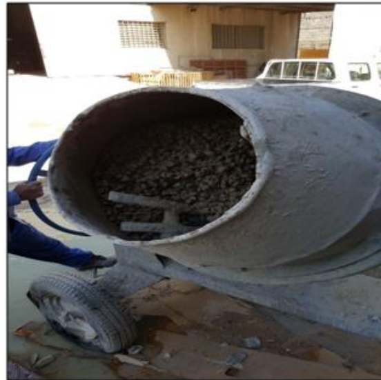
Figure 3.13 Adding BMF Inside the Concrete Mechanical Mixer
