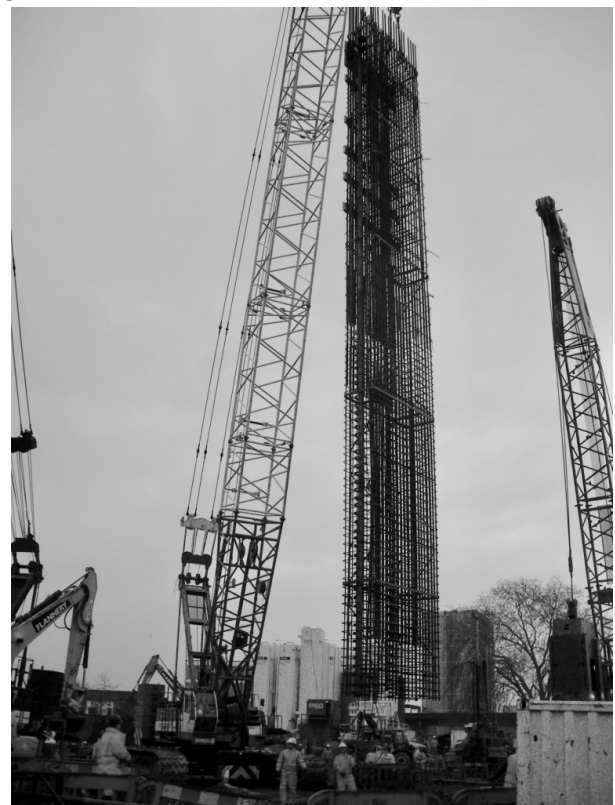
Figure 4 Installation of instrumented reinforcement cage
