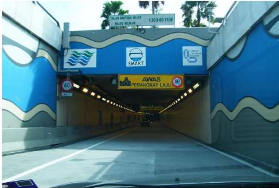
Entering the SMART flood tunnel, Kuala Lumpur, Malaysia. Photo: flickr.com/photos/emrankl/
