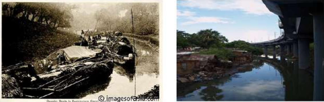
Figure 86: Buckingham canal in early 1900's(left) and Buckingham canal with MRTS line running over it and slum settlements below(present time).Source- Studies and Research related to Cooum Sivakolundu,, National Institute of Ocean Technology, Chennai
