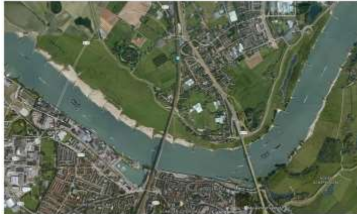
Before: Dikes on the north shore of the River Waal (seen as a roughly U-shaped squiggly line) come close to the river itself, creating a water bottleneck and flood risk during heavy rains. (Google Maps)
