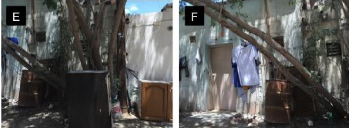
Figure 59: Unplanned vegetation in the houses of Najma, 2016. Source: Author
