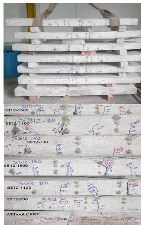
Figure 8. Crack pattern of RC slabs strengthened with CFRP under the four-point bending test.
