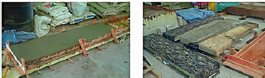
Figure 5. Schematic of casting and curing of the prepared slabs.
